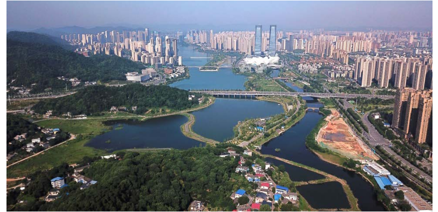
Smart Water Project (Phase I) of Longwang Port Basin in Xiangjiang New District, Hunan Province
