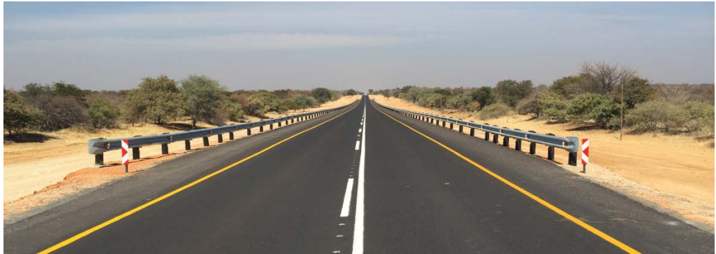
The Upgrading to Bitumen Standard of Main Road 67 Between Omakange and Ruacana,Namibia
