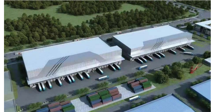
Beijing Qianxi Crane Cold Chain Logistics Project
