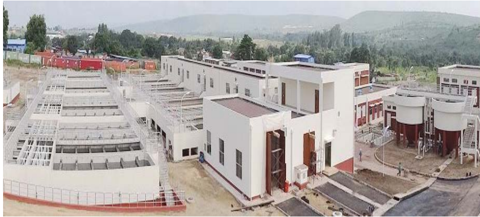
Djiri Drinking Water Treatment Plant Project, Congo(Brazzaville)
