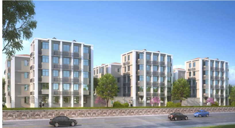
Renovation of Old Residential Communities in Beijing
