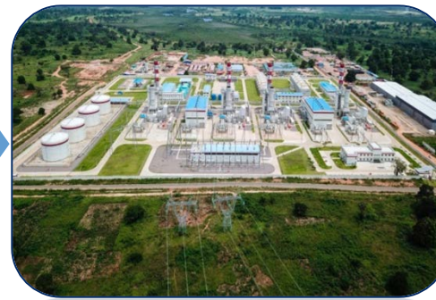
Soyo I Combined Cycle Power Plant
