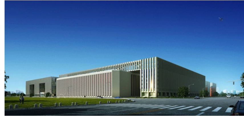
Tencent Internet Data Center Project
