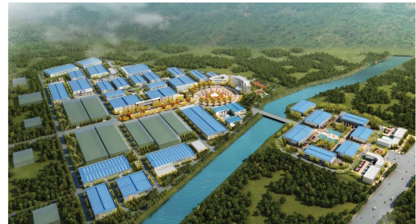
CRRC Yongji Intelligent Manufacturing Logistics Park
