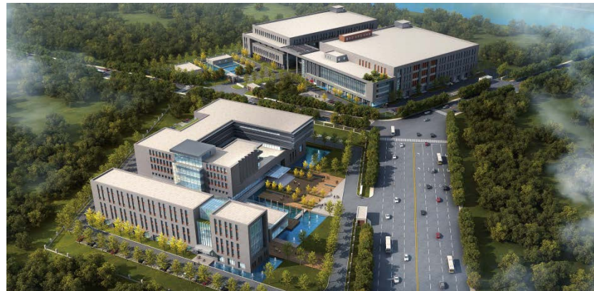
TianJin Ultra-micro Filtration Membrane Project with Annual Output of 1245 Tons
