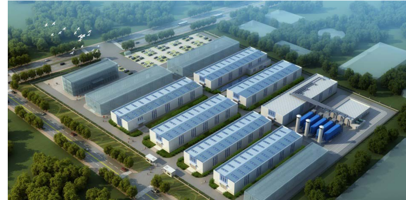
ETI Mine-Bandirma Boron Carbide Production Plant Project, Turkey
