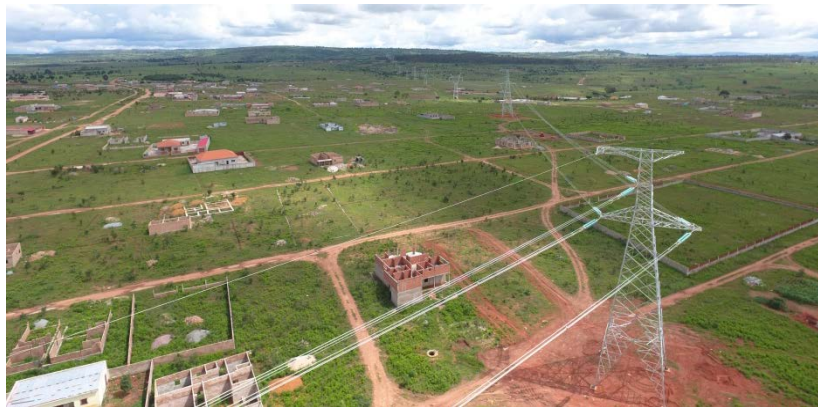
Lauca 400kV Transmission Line Project, Angola
