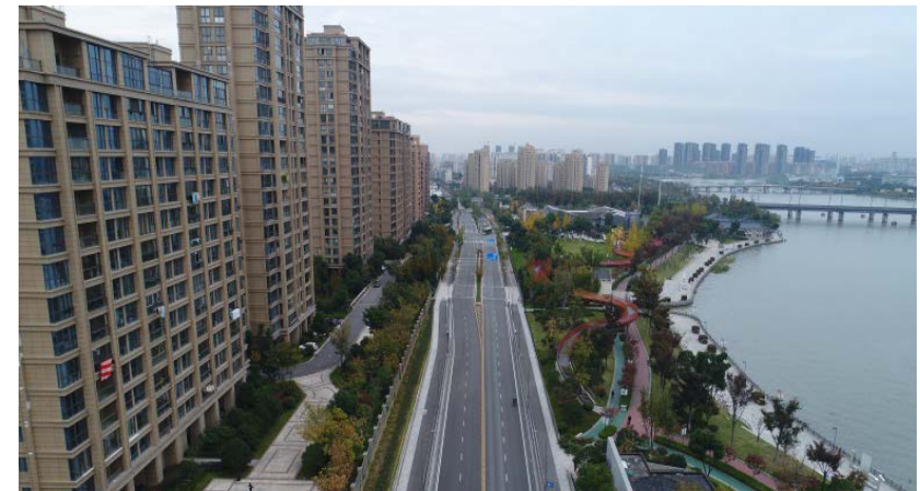
Sponge Renovation Project in Xiejia and Tianshui District of Ningbo City
