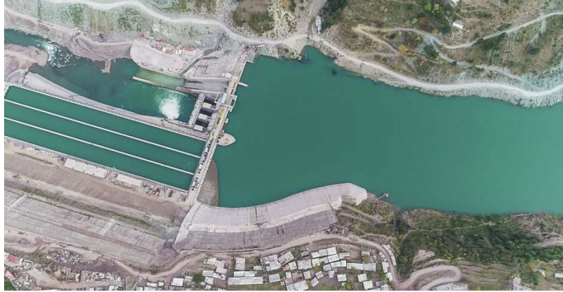
Neelum - Jhelum Hydro electric Project,Pakistan
