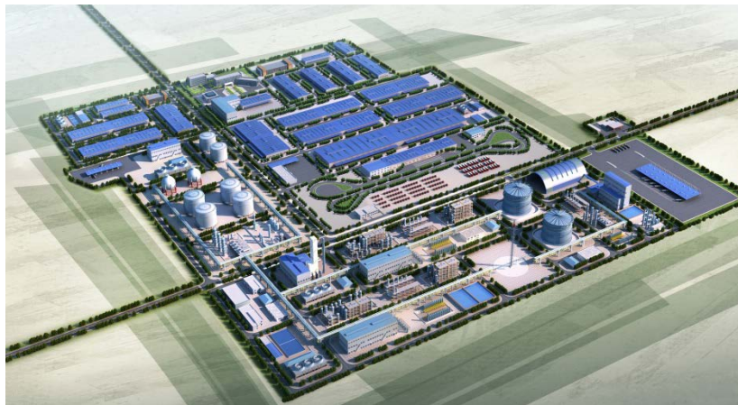
Shanxi Pengwan Qinggang Hydrogen Production (20,000t/yr) from COG Project
