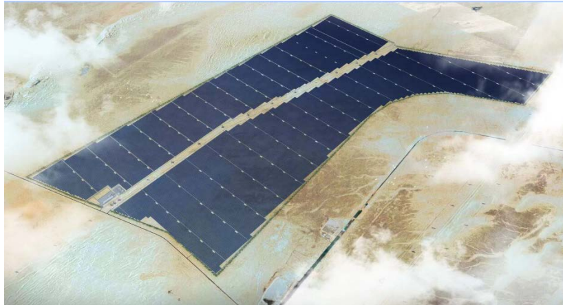
Al Dhafra PV2 Solar Power Plant,UAE
