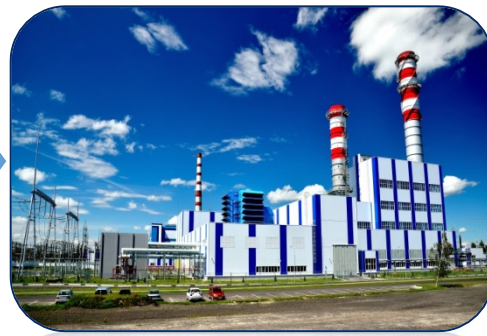
Berezovskaya 427 MW Combined Cycle Power Plant
