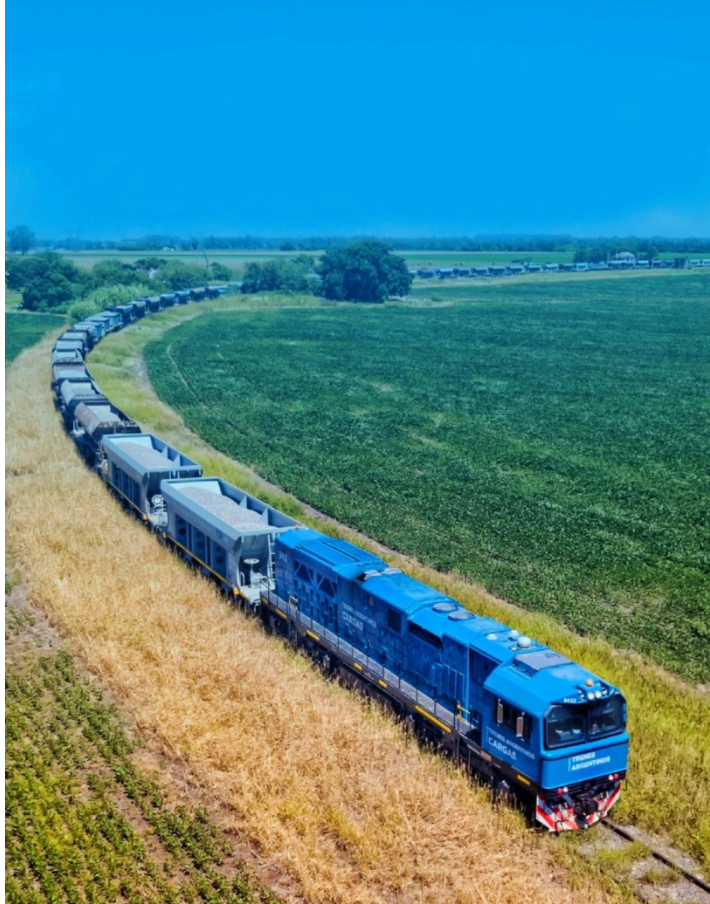
Belgrano Cargo Railway Rehabilitation Project in Argentina,Argentina
