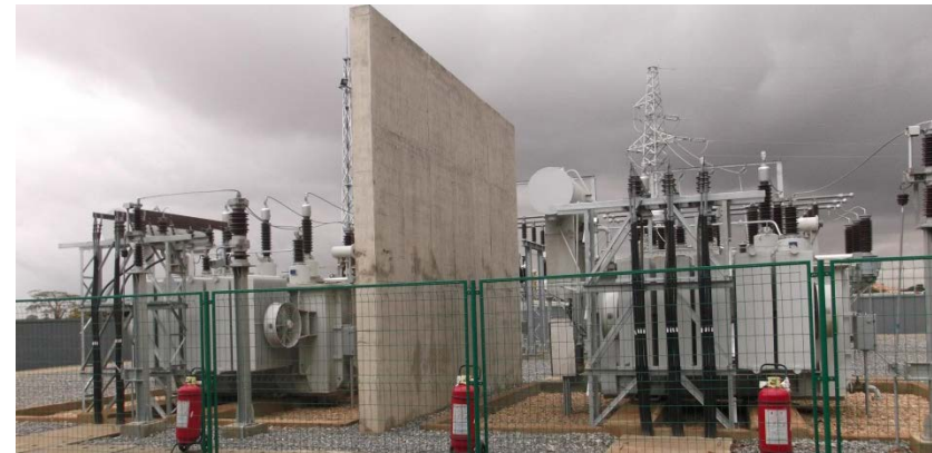
Rehabilitation and Expansion of the Luanda Electricity Network Project, Angola
