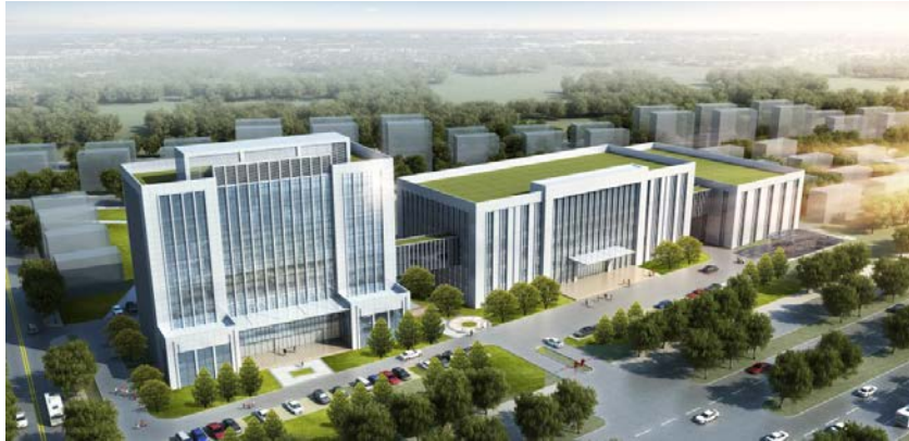
China Unicom Hengyang Big Data center
