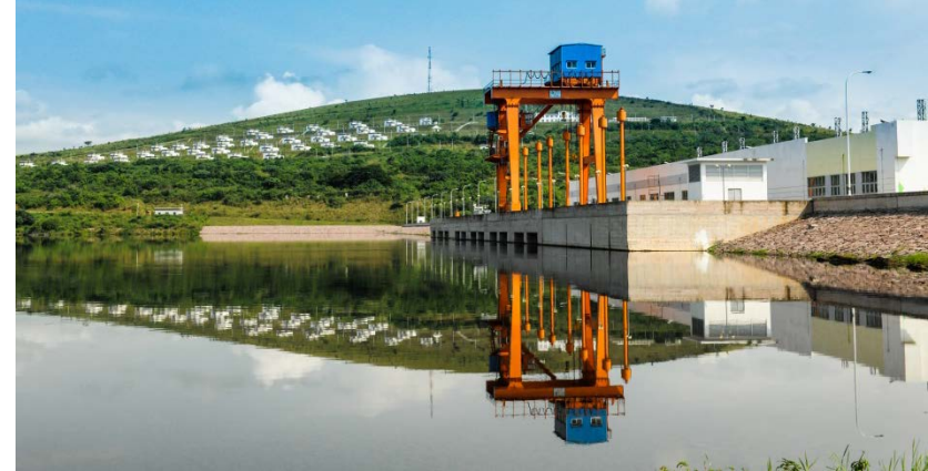
Imboulou Hydropower Plant ,Congo(Brazzaville)
