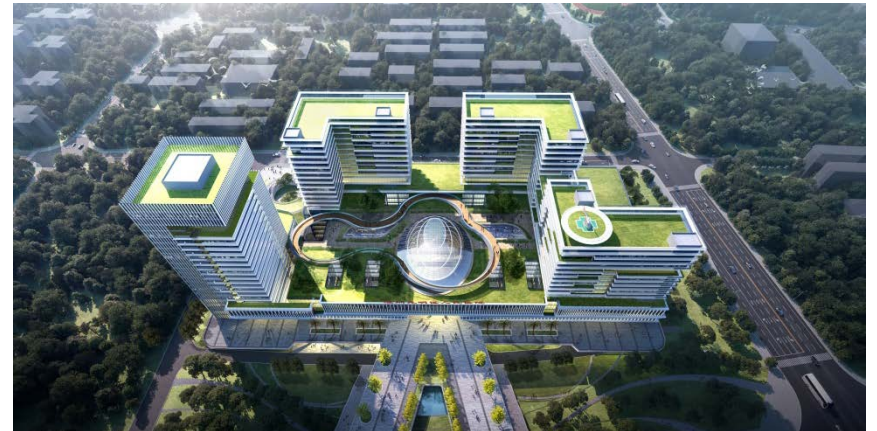
New Setting of Guangming District People's Hospital in Shenzhen
