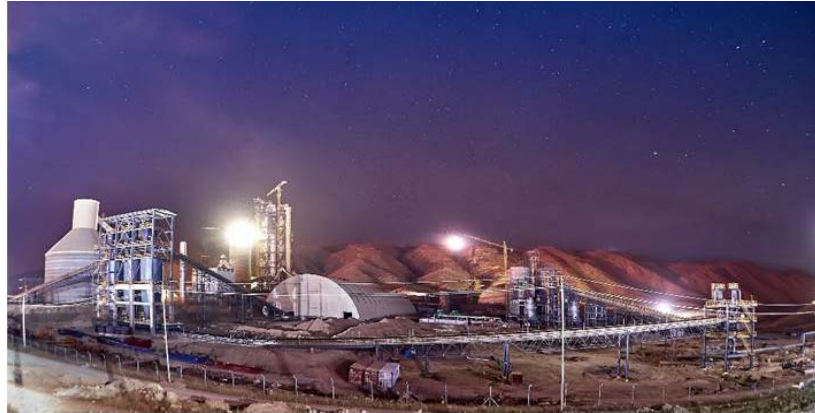
KAR Group Cement Plant in Qarachog, Iraq
