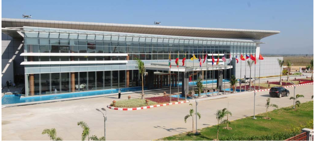
Nay Pyi Taw International Airport Project,Myanmar
